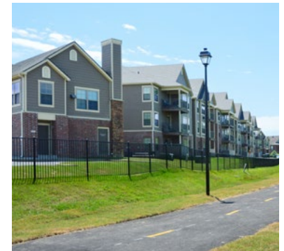
Multi-use structures facing a shared use path.
