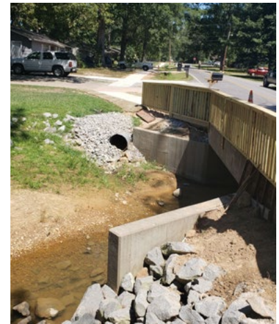
Box culvert with sidewalk.
