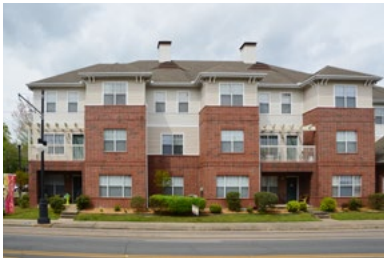
Apartment building with building articulation, including balconies.
