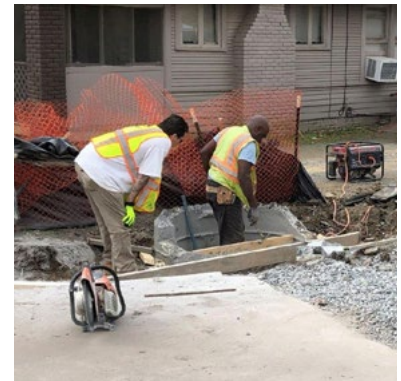
Drainage improvements under construction.
