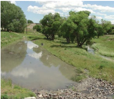
Detention ponds hold water for a short period of time; this pond temporarily holds water before it enters the stream. Photo: https://www.lccdnet.org/wp-content/uploads/Ponds.pdf
