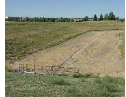
On-channel detention ponds reduce peak storm flows and provide flood control for downstream neighborhoods. Photo: https://www.lccdnet.org/wp-content/uploads/Ponds.pdf
