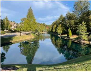
Retention ponds maintain a pool of water throughout the year and hold stormwater runoff following storms.
