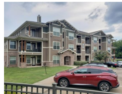
This multi-family development was constructed as a PUD on a large parcel, and includes amenities such as a swimming pool and a dog park.
