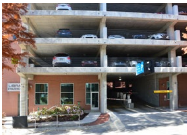
A parking deck.
