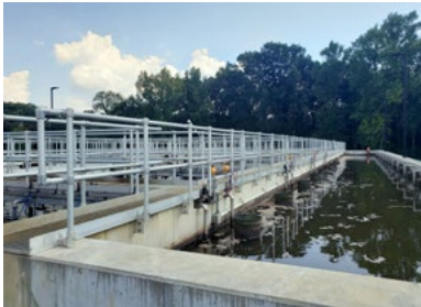
Wastewater treatment facility.
