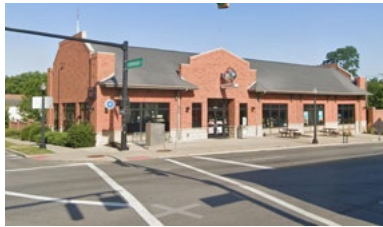
These gas stations’ primary buildings are built close to the street corner.
