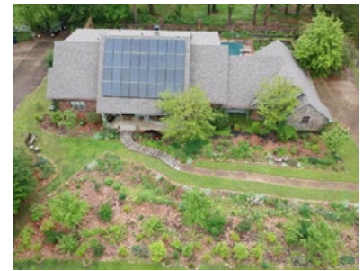
Roof-mounted solar panels. Photo: Layet Johnson
