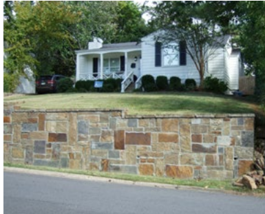
A retaining wall.
