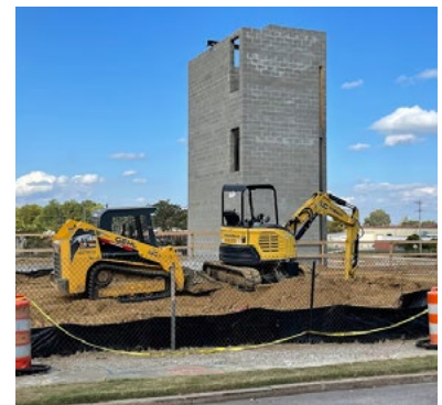
A commercial building under construction.
