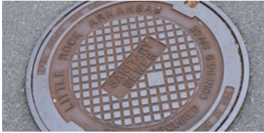
A sewer manhole cover.
