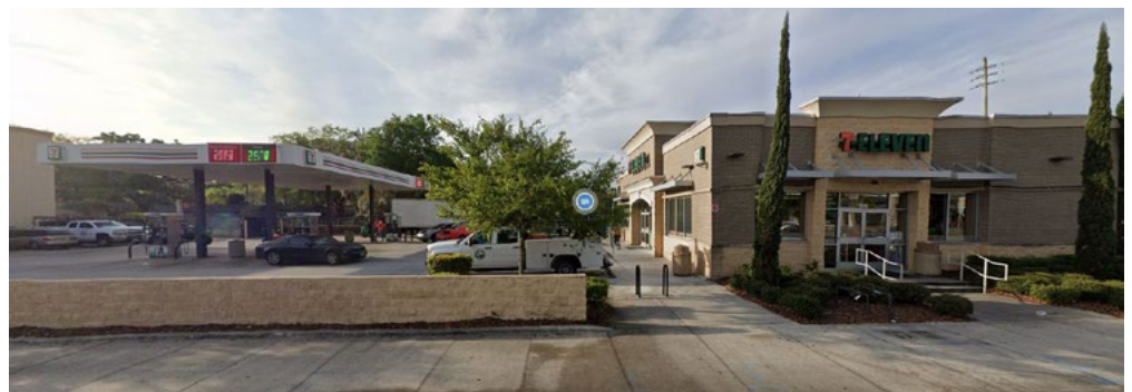
Gas canopies behind a garden wall.
