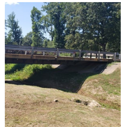
Bridge over a drainage path.
