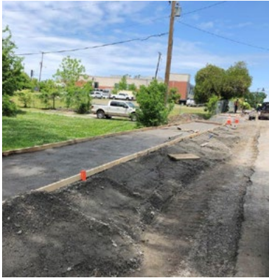
A roadway and sidewalk under construction.
